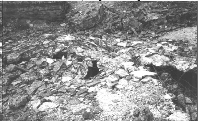
Photo 31: Concrete roof of morgue 1 of crematorium II in Birkenau in August 2000. Opening 8 (in the center) and continuation of crack (see photo 30), of which opening 8 is a part.
