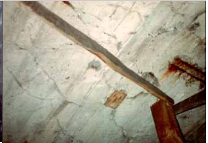
Document 10: Another one of the supporting blocks for lamps in the ceiling of morgue 1 of crematorium II at Birkenau. October 1991. © Carlo Mattogno.
