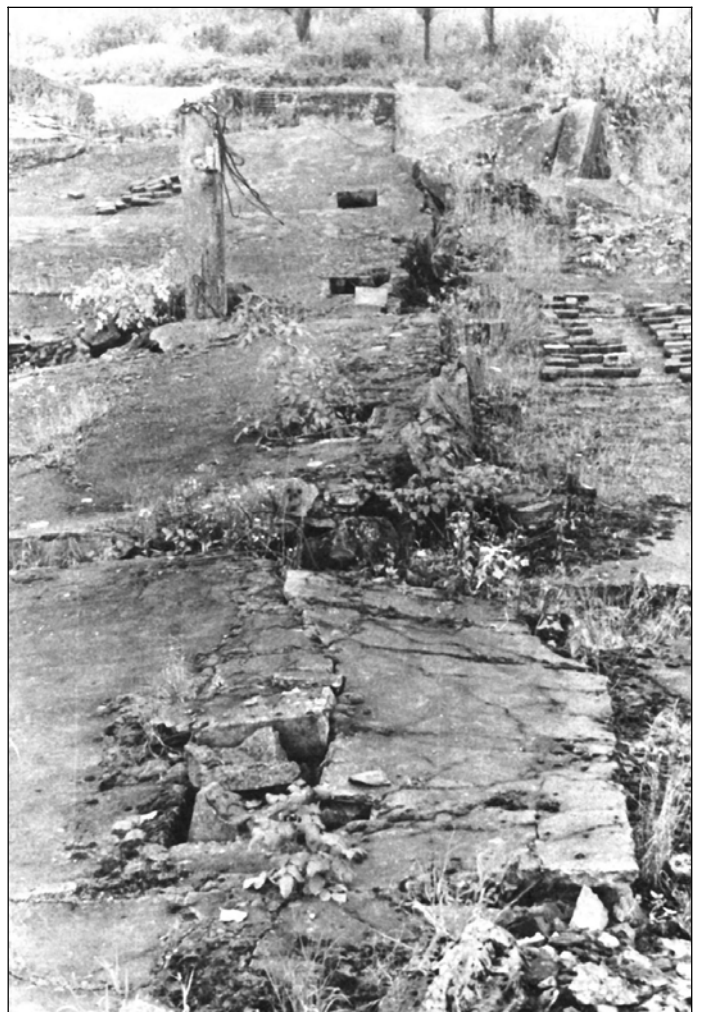
Photo 11: All five ventilation openings of the ceiling of the oven room of crematorium III. Photo by J.-C. Pressac.
