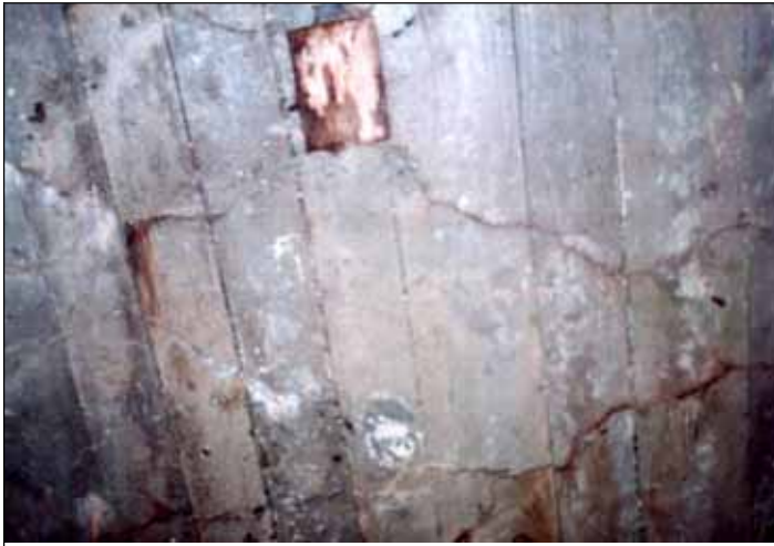
Document 9: One of the supporting blocks for lamps in the ceiling of morgue 1 of crematorium II at Birkenau. October 1991. © Carlo Mattogno.
