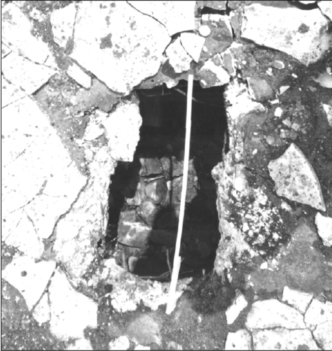
Photo 15: Concrete roof of morgue 1 of crematorium II in Birkenau. Opening 2 in August 1997. © Carlo Mattogno
