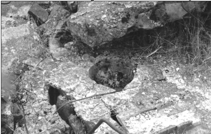
Photo 8: Round opening for the pipe of the ventilation through the reinforced concrete roof of morgue 2 of crematorium II in Birkenau. October 1991. © Carlo Mattogno
