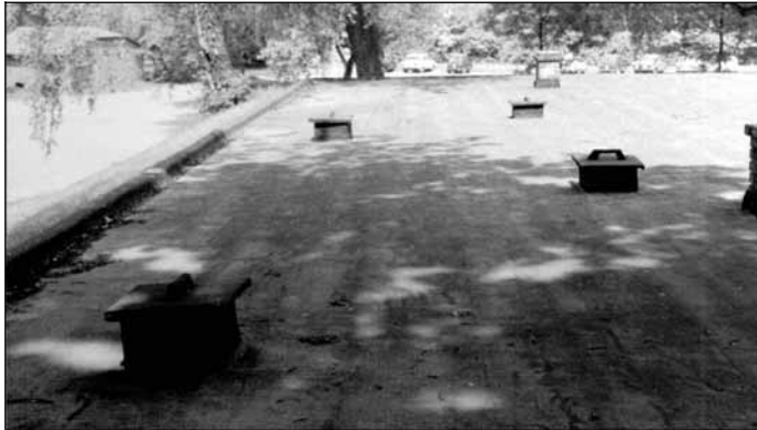
Document 11: Photo of the roof of the morgue. All four shafts constructed by the Poles after the war. © Carlo Mattogno.
