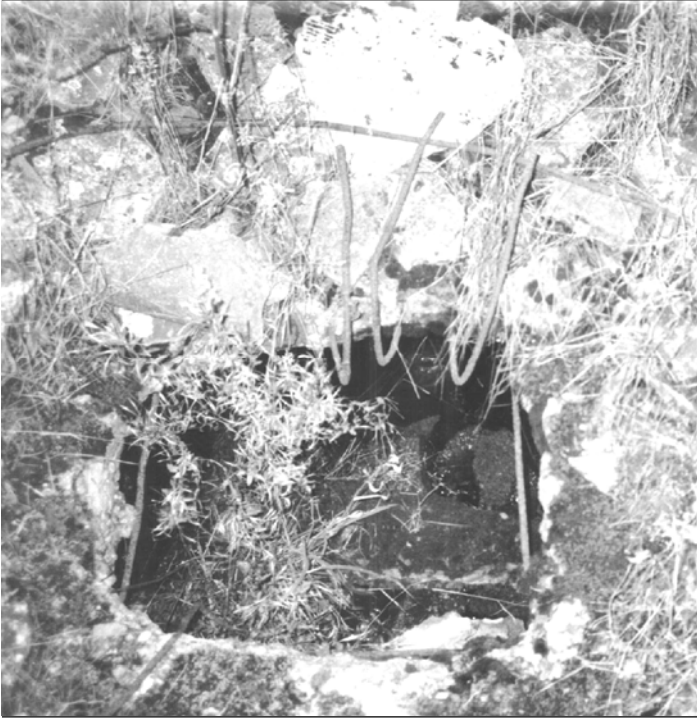
Photo 22: Concrete roof of morgue 1 of crematorium II in Birkenau. Opening 7 in October 1991. © Carlo Mattogno
