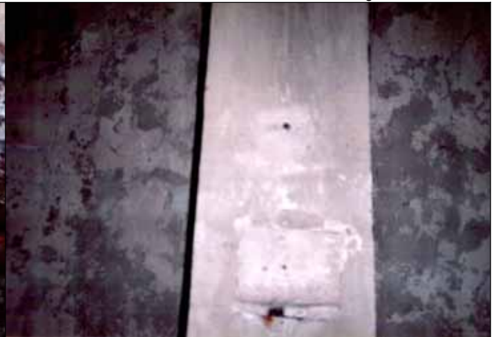
Document 12: Morgue of crematorium I at Auschwitz. One of the blocks set into the center of the supporting beam of the ceiling. October 1991. © Carlo Mattogno.
